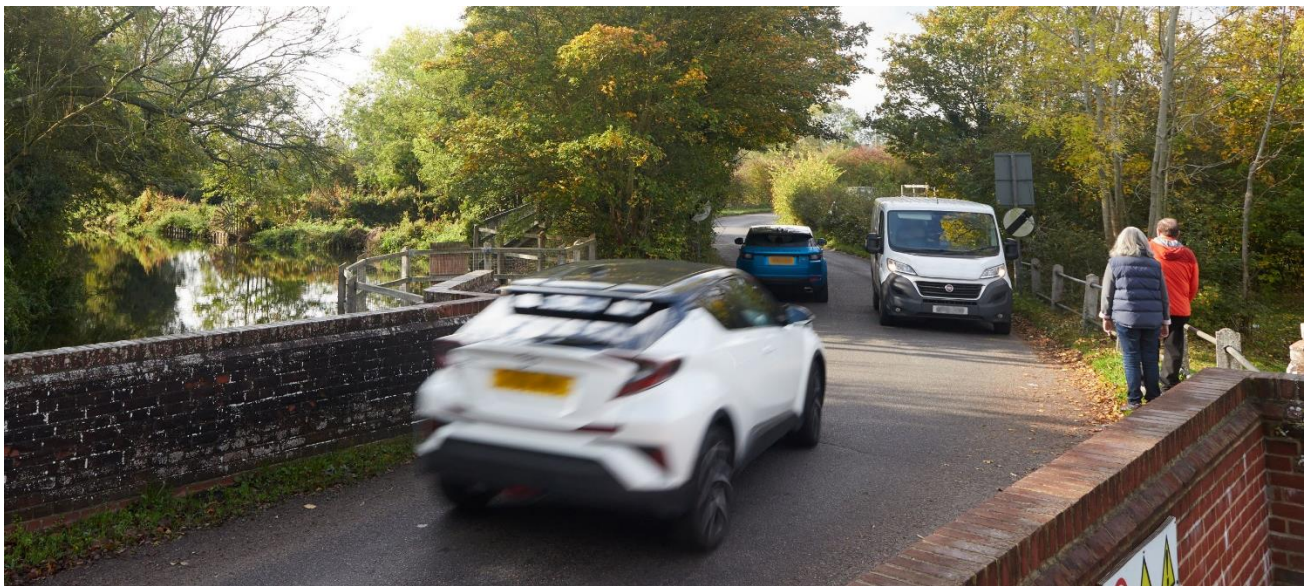
Figure 2-15 - Costessey Lane Bridge
